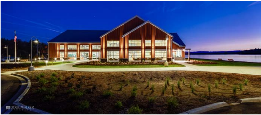
Kalama Interpretive Center, as delivered to client
